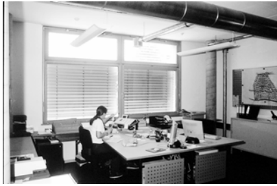
Figure 2: Split exterior blinds allow the occupant to prevent direct glare through the lower section (shown closed) while lighting the office with daylight through the upper section (shown partly closed). Photo © Fraunhofer ISE, 2001.
