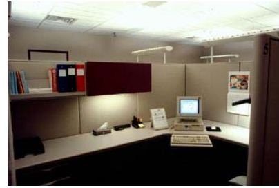
Figure 3: One way to deliver bright light to where it will be seen is to use a task-ambient combination, with areas of high illuminance provided locally by task lighting. Photo © 1996, National Research Council Canada.
